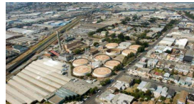
Wastewater treatment has several stages and requires large facilities
