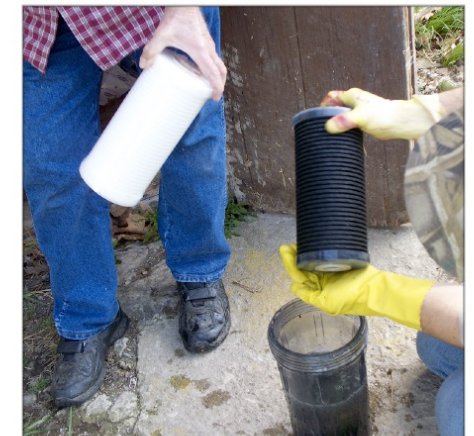
"The Changing of the Water Filter"
